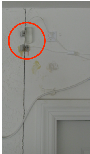
Interface Crack
